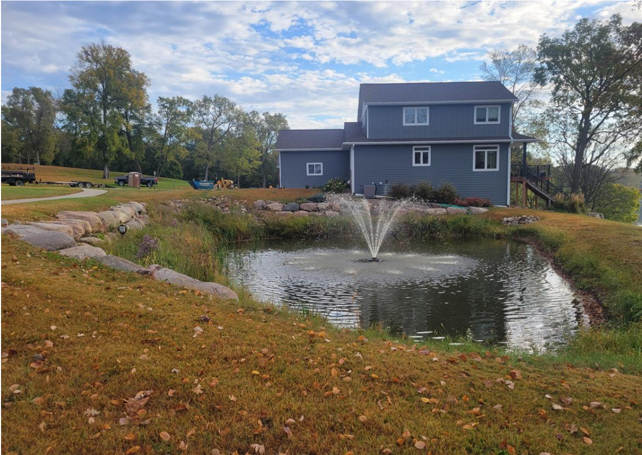
Existing stormwater pond
