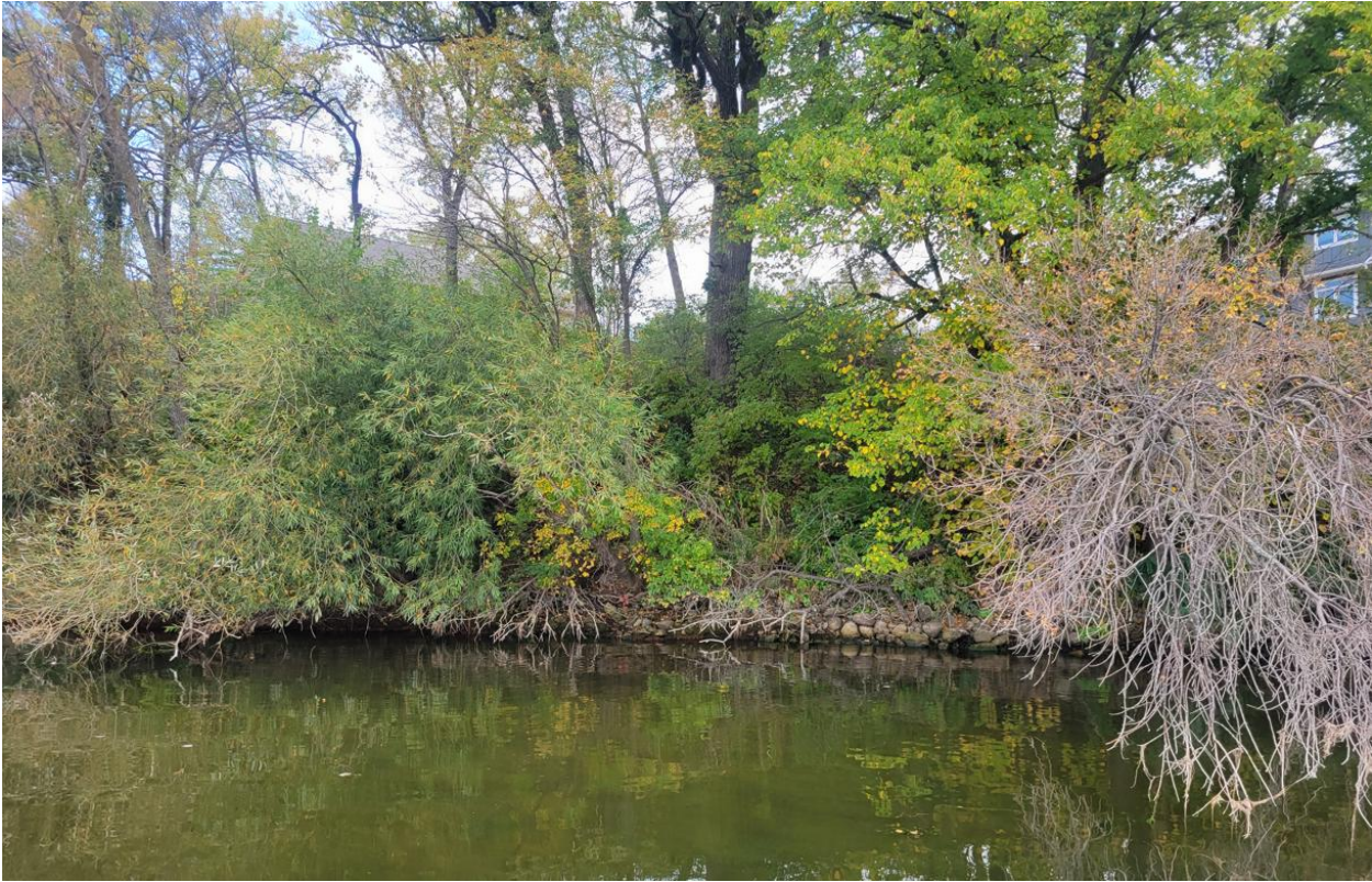
Typical stable bluff toe along Lake Koronis. Note mature vegetation and rock toe.
